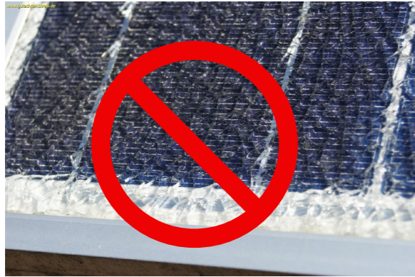
Broken glass, damage probably caused by impact, for example hail, stones etc. 11
