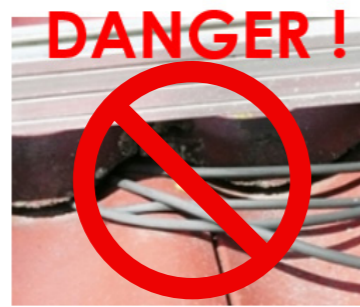
Improper cable installation 13
